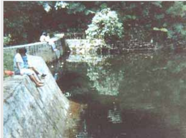
Yerba Buena's finished dam and water supply
